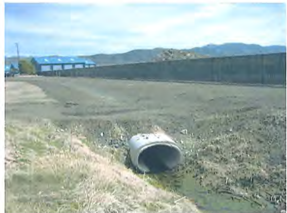
Ex. Paving and Ditch Conditions
