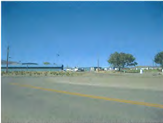
View of Corp Yard Sheds, Facing Northeast
