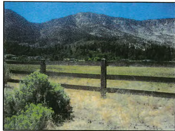
Concrete Railing Example
