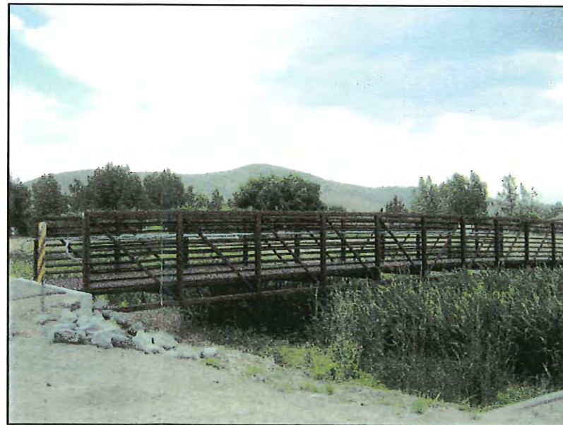
Existing Metal Bridge off Saliman Street
